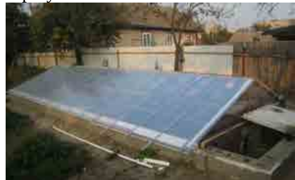
b) an underground pit of two-leaf greenhouse
