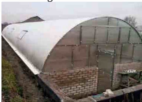
c) the arched or tunnel greenhouse-thermos
